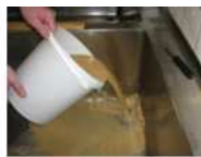
Component 2 distributed into the same drains as component 1 beforehand
